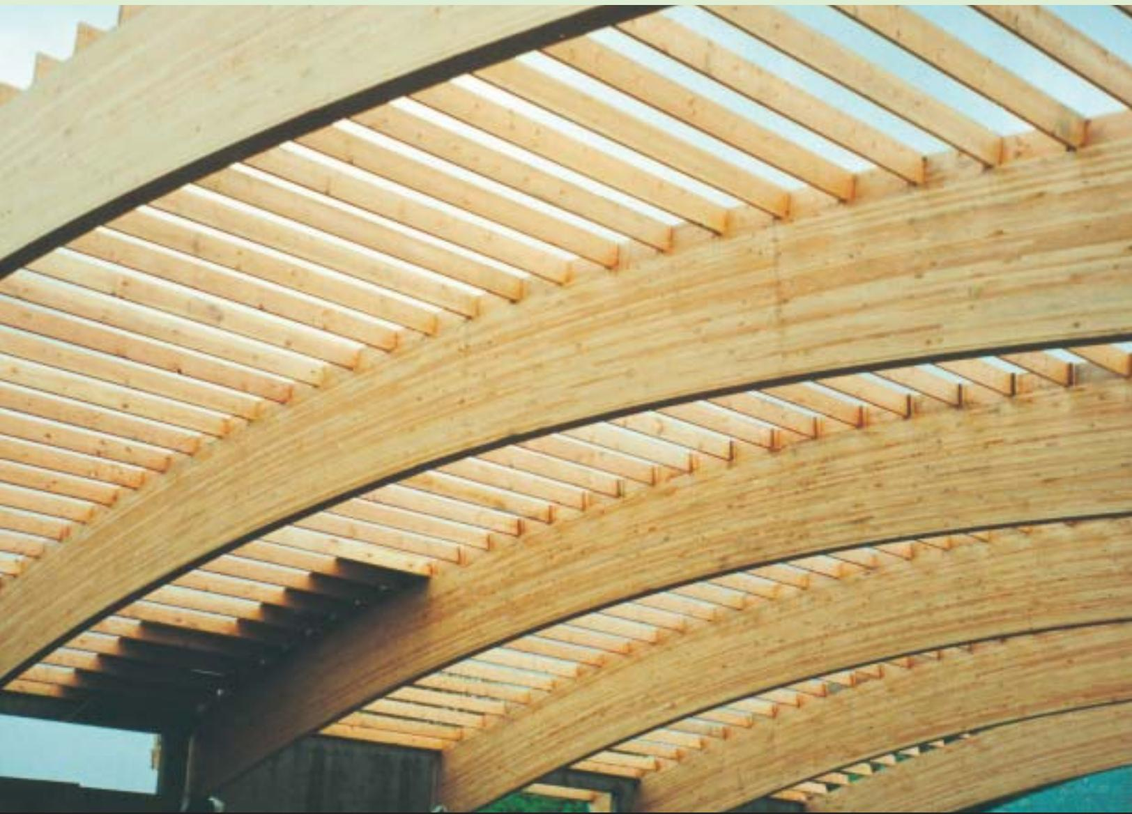
*Engineered wood products allow long span capability while retaining the aesthetic appeal and environmental advantage of wood construction.*
